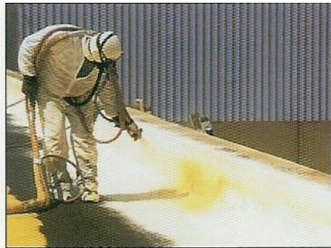
Foam & Coatings System for existing BUR Asphalt Roofs
